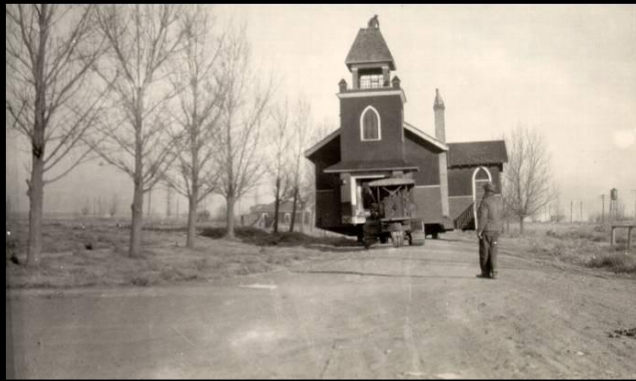
Figure [5] – A historic photo of a church being moved. 179 The basic “how to” was to raise the structures up on logs and then pull the logs with a tractor or other machinery. 180
