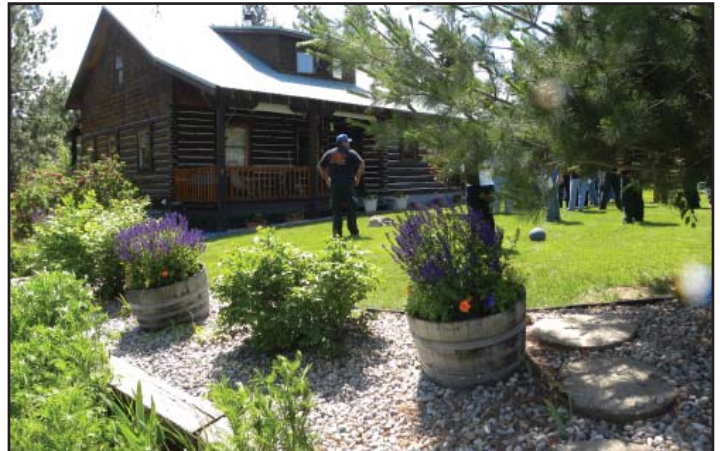
Consider replacing flammable mulches with nonflammable materials such as rock or gravel.
