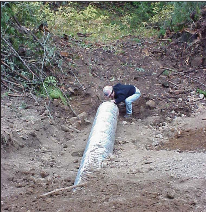
Culvert inspection. Photo by R. Barkley, Idaho Department of Lands.
