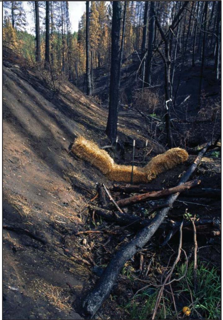
Straw bale check dam.
