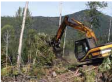
Figure 32. Excavators can separate fine from coarse woody debris more easily.
