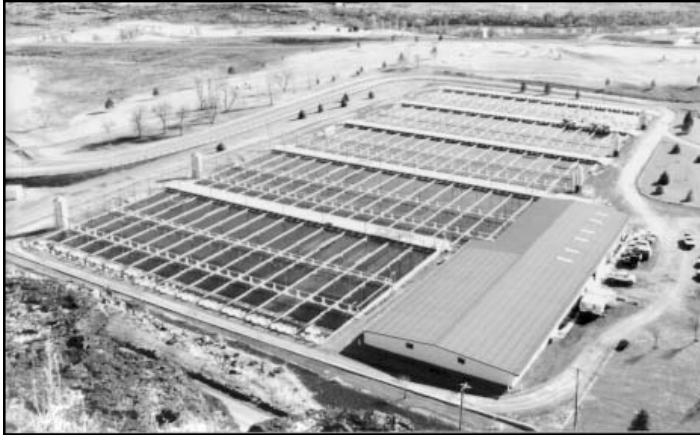
Figure 7.1: Raceways used for trout production.
