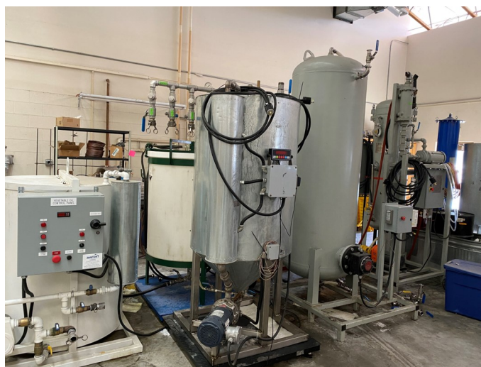
The biodiesel facility at J.W. Martin lab is being decommissioned
