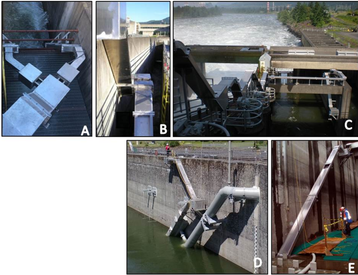
Figure 2. A) Bradford Island LPS two collector ramps; B) Washington Shore LPS two collector ramps; C) Cascades Island LPS collector ramp; D) Washington Shore Fishway LPS vertical collector, closed tube with baffled opening collector, Lamprey Flume Structure; E) John Day bollard field (foreground) and open ramp LPS collector.
