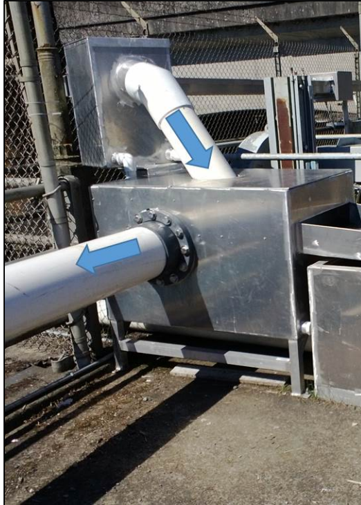
Figure 11. The pond feature of the CILPS. The arrows indicate the direction of fish movement through the box. The lamprey first encounter an upwelling box (upper left) that receives water pumped up from the pond (large aluminum tank in center of photo). Lamprey drop from the upwelling box into the pond and then volitionally enter the PVC exit pipe that leads them to the structure terminus and exit slide. The pond can be closed off from the PVC exit slide if the structure is to be operated as a trap.
